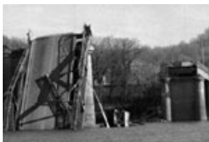
Silver Bridge after collapse
